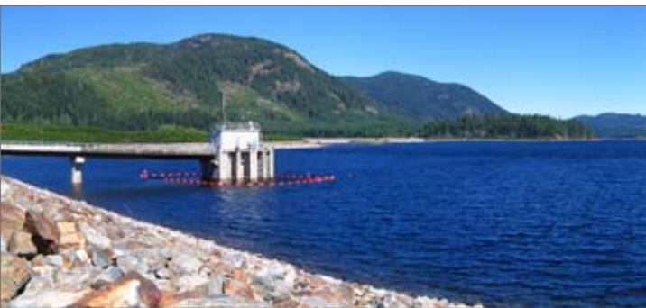
Water Intake Tower at Sooke Reservoir.
