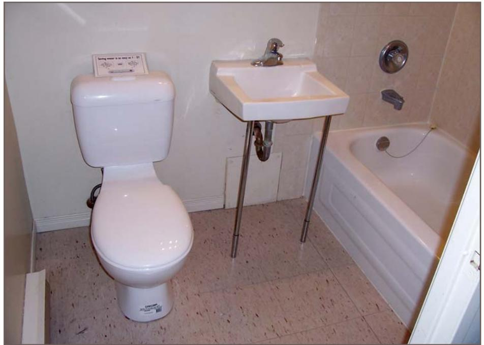
Figure 5—The high-efficiency (HET) Caroma dual-flush toilet used for this project. It uses three litres of water to flush liquid waste and six litres to flush solid waste.
