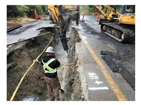
Figure 21 – Residual Solids Conveyance Line - Hoe ramming bedrock around water service at Grange Road.
