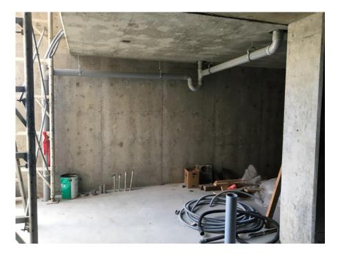
Figure 11 – Clover Point Pump Station – forming walls and column
