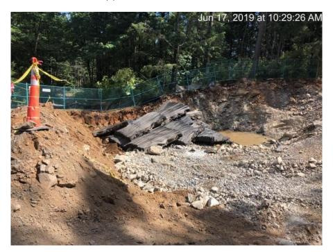
Figure 23 – Residual Solids Conveyance Line': Blast matts in place prior to blast #1 at pump station #3
