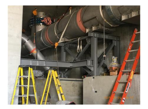
Figure 5 – Mcloughlin Point Wastewater Treatment Plant – installing pipe supports for backwash water header.
