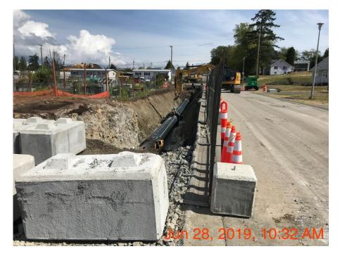
Figure 13 – Macaulay Point pump station & forcemain – completing an in ditch fusion weld at Anson Street..
