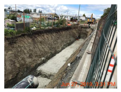
Figure 14 – Macaulay Point pump station & forcemain – Forcemain bedding compaction in progress.
