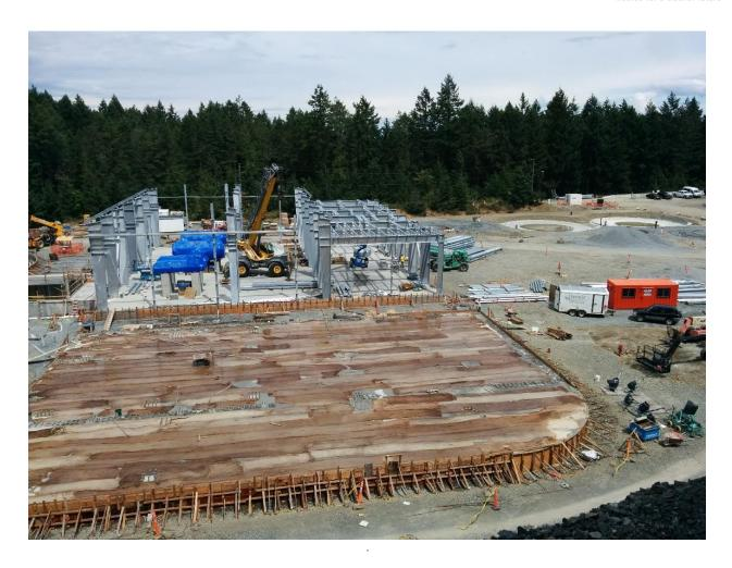
Figure 8– Residuals Treatment Facility – Dry building foundation wet curing and steel erection of Residuals Handling Building.
