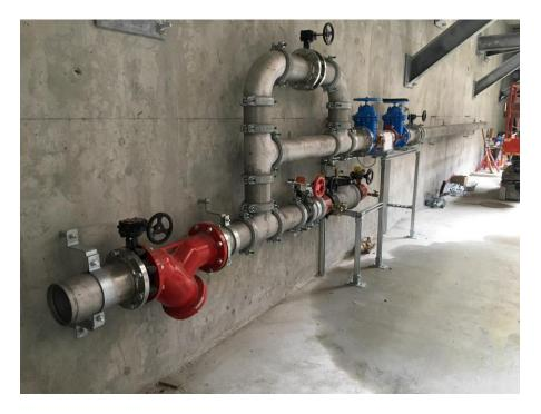
Figure 9–Clover Point Pump Station – installation of water entry piping in the pump room
