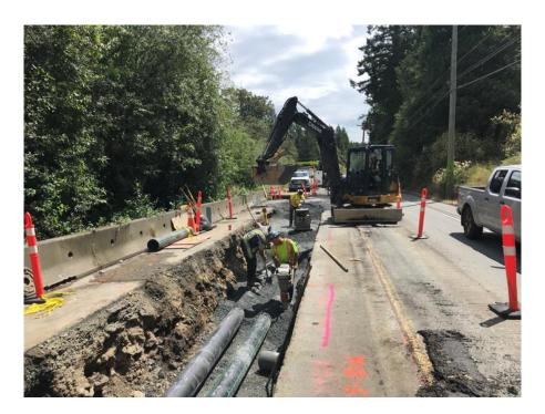
Figure 20 – Residual Solids Conveyance Line: Bedding and backfilling pipe at Interurban Road.
