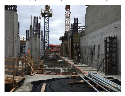
Figure 2 – Mcloughlin Point Wastewater Treatment Plant – Forming columns in Operations & Maintenance breeze way.
