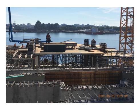
Figure 4 – Mcloughlin Point Wastewater Treatment Plant – decking of Biological Aerated Filter heat recovery room suspended slab.
