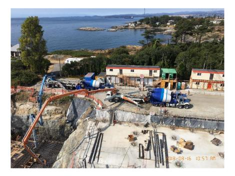
Figure 6 – Placing concrete in the tertiary slab.
