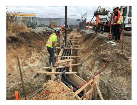
Figure 19 – Placing concrete in duct bank under View Point Road.
