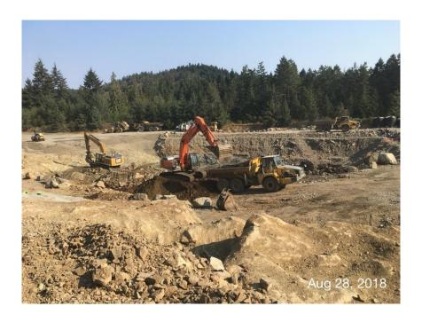
Figure 12 – Loading and hauling contaminated material to Hartland Landfill.
