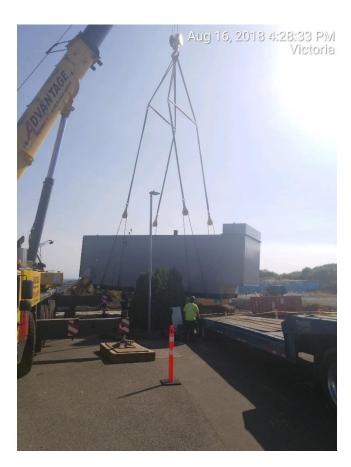
Figure 18 – Hoisting E-house and moving to new location.
