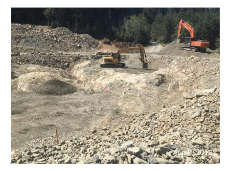
Figure 11 – Excavator with hoe-pack compacting placed aggregate material in valleys and depressions in bedrock.
