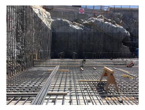
Figure 2 – Rebar dowels in the tertiary area.
