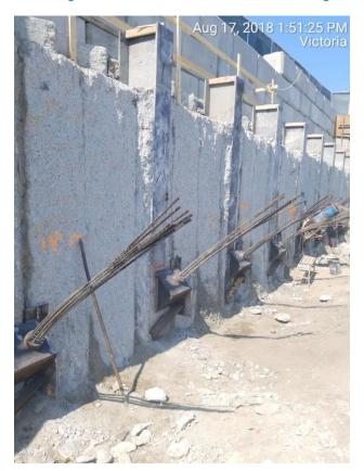
Figure 17 – Tension and proof testing tie-backs.
