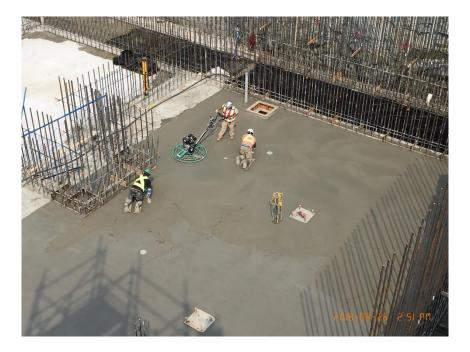
Figure 8 – Finishing concrete in the tertiary slab.
