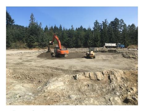
Figure 10 – Spreading and compacting aggregate at digester #1 location.
