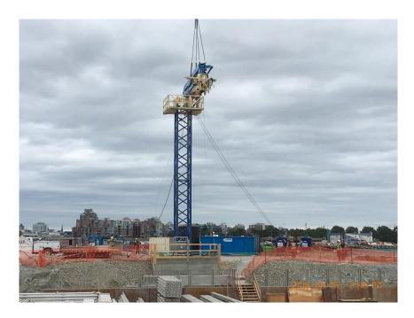
Figure 3- Erecting concrete placing boom for operations and maintenance (O&M) area.
