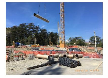
Figure 2 – Staging of under slab BAF piping
