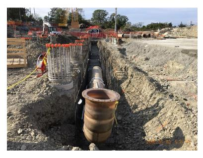
Figure 3- Installation of under slab pipe
