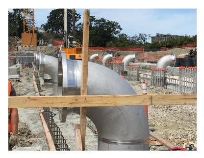
Figure 8 – Install & align stainless steel risers in West BAF drain
