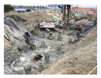
Figure 4 – Installation of foundation piles in odour control area
