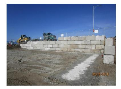
Figure 9 – Installation of guide wall and preparation of drill pad and retaining walls
