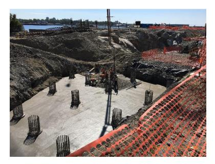
Figure 6 – Placing concrete mud slab in odour control area
