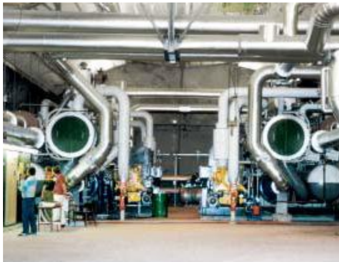
Figure 2 Installation of Two (6.5 MW) Heat Pumps with Shell and Tube Heat Exchangers for Heat Recovery From Raw Wastewater (Note: raw wastewater is subject to mechanical screening and sedimentation prior to use) (Source: Friothersm, 2005)
