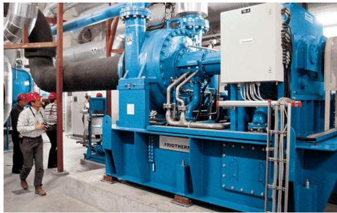
Figure 2 Installation of Two (6.5 MW) Heat Pumps with Shell and Tube Heat Exchangers for Heat Recovery From Raw Wastewater (Note: raw wastewater is subject to mechanical screening and sedimentation prior to use) (Source: Friothersm, 2005)
