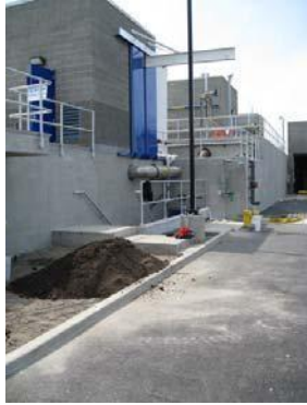
Hoist for Sand Storage
