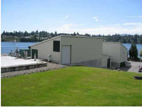
Storage Tank, Actiflo Building and Chemical Building
