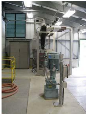
Inside Actiflo Building
