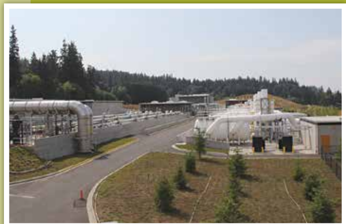
A bird's eye view of Seattle's Brightwater wastewater treatment facility.
