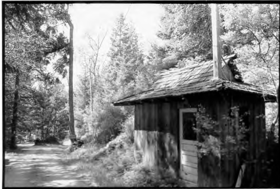
HIGH HILL PUMP HOUSE AND ROAD photo: M. Levy
