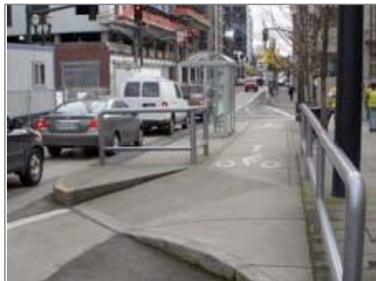
Figure 5. Pavement markings direct bicyclists onto the streetcar platform from the bicycle lane.
