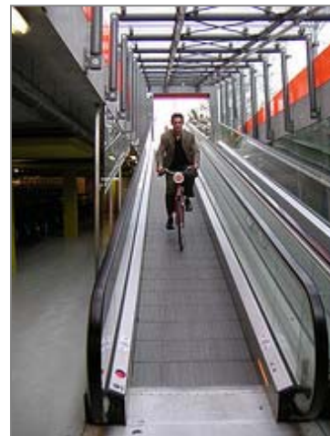
Figure 3. Bicycle Escalator at a Bicycle Parking Garage in Amsterdam
