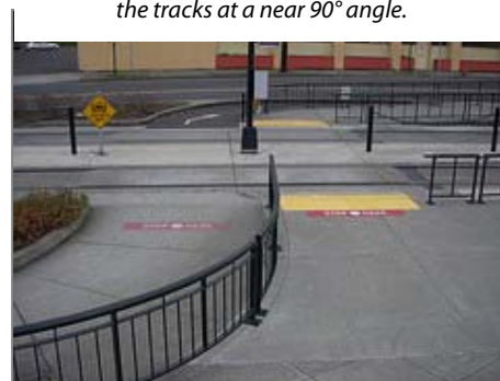
Figure 7. Fencing and pavement markings direct bicyclists to cross streetcar tracks at a 90° angle.
