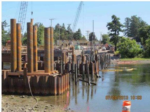
Photo 7-3 Existing bridge deck removed and caisson installation initiated.
