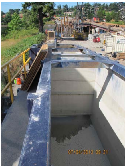
Photo 9.15-1 Silt-laden water treatment tank prior to filling.
