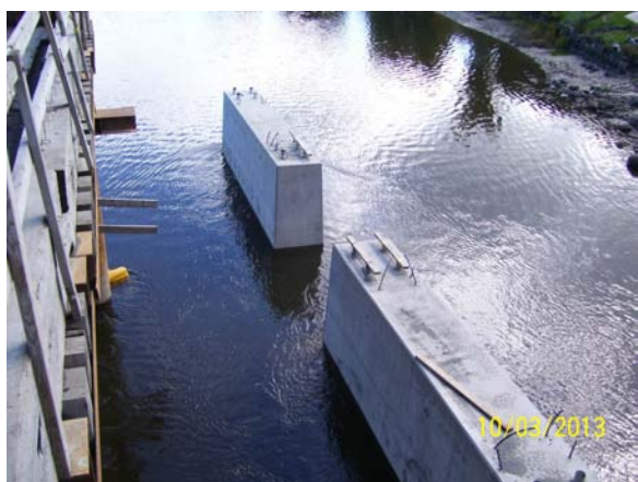
Photo 8-3 Completed south piers with the sheet piling removed.
