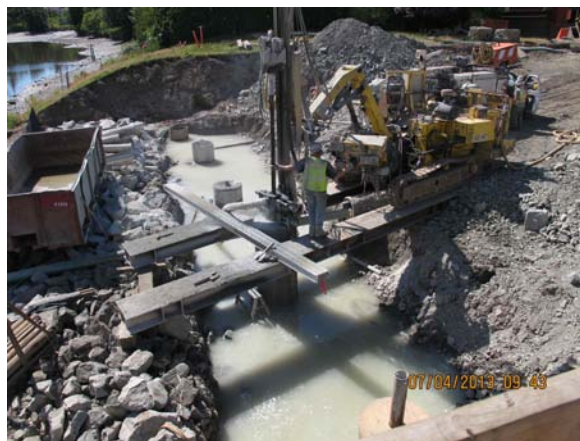
Photo 9.17-1 Contained concrete slurry during construction of the south abutment.
