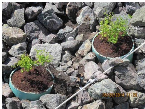
Photo 11.3-6 Planting wells in riprap on southeast quadrant.
