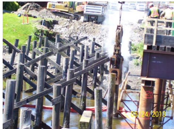
Photo 7-4 Vibratory hammer used to remove creosote timber piles.
