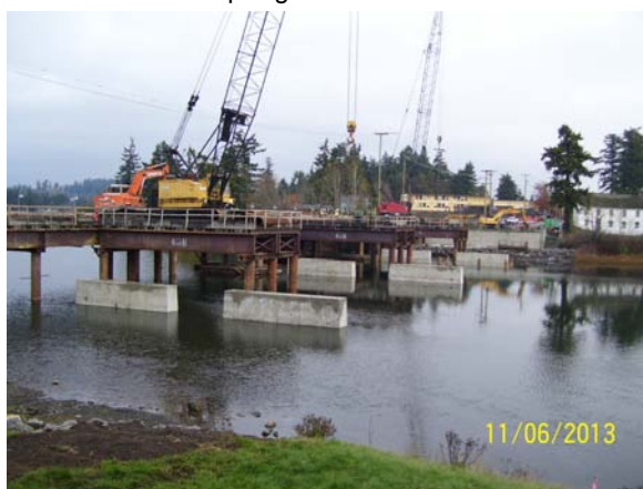
Photo 8-4 All three sets of piers complete and ready for bridge erection.
