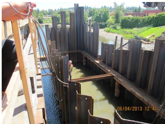
Photo 8-2 Sheet piling around the south caisson.
