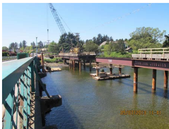
Photo 6-2 Work bridge construction.
