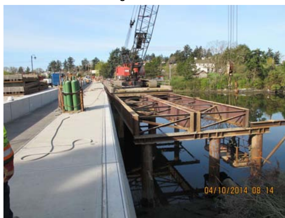
Photo 6-4 Work bridge dismantling adjacent to the replacement bridge.
