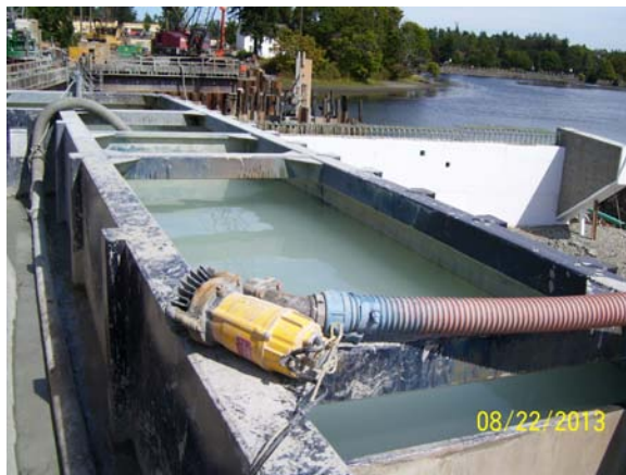
Photo 9.15-2 Operational water treatment tank.
