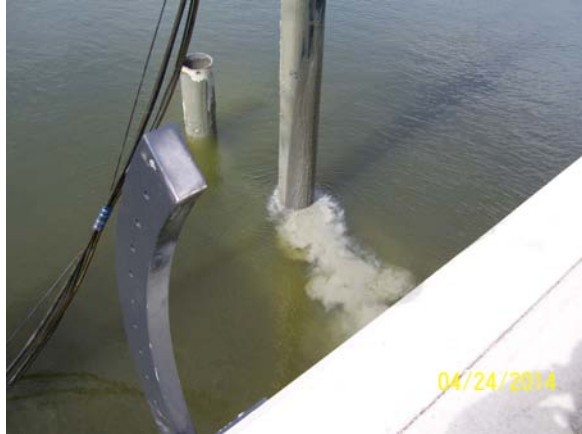
Photo 10.2-1 Sediment release during temporary work bridge pile pulling.
