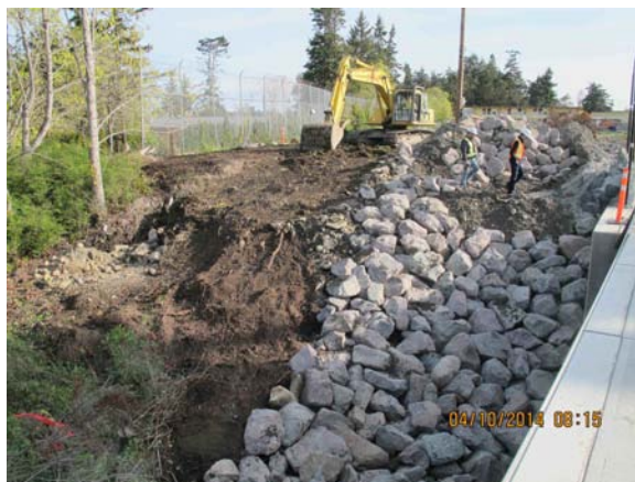
Photo 11.3-1 Preparation of the northwest quadrant bank for riparian planting.
