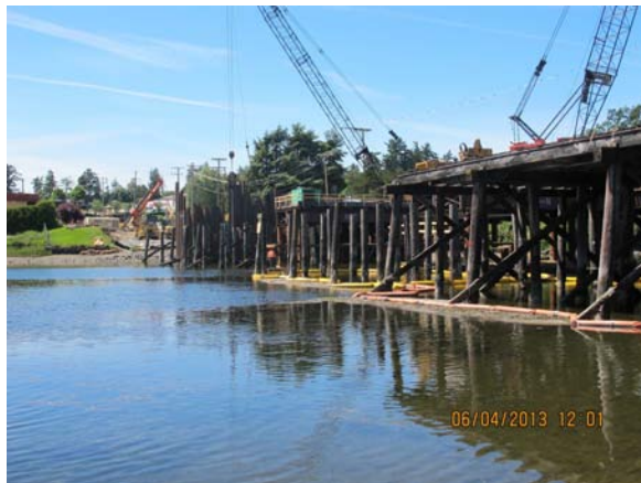
Photo 7-1 Existing Craigflower Bridge demolition.
