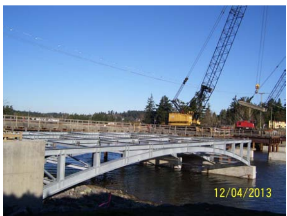
Photo 8-5 Placement of the south girders.
