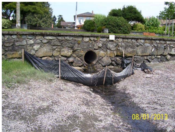
Photo 10.4-1 Storm outfall containment.
