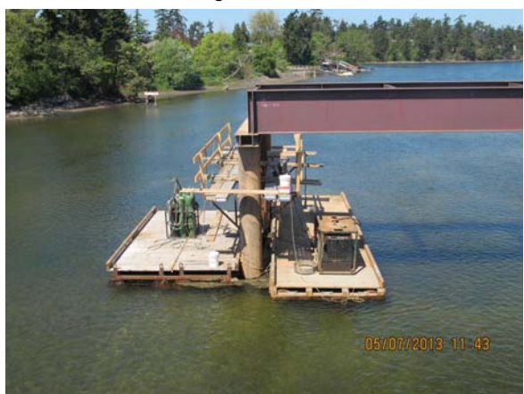
Photo 6-3 Work bridge construction.
