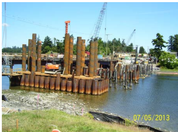
Photo 8-1 Installation of the first and second caissons.
