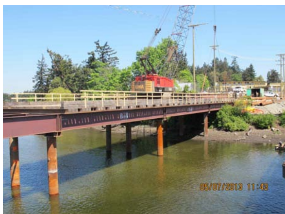
Photo 6-1 Work bridge construction.
