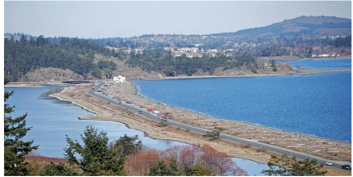
Image 2: The Esquimalt Lagoon spit, illustrating the road and eroding beach. (Capital Regional District, 2013)
