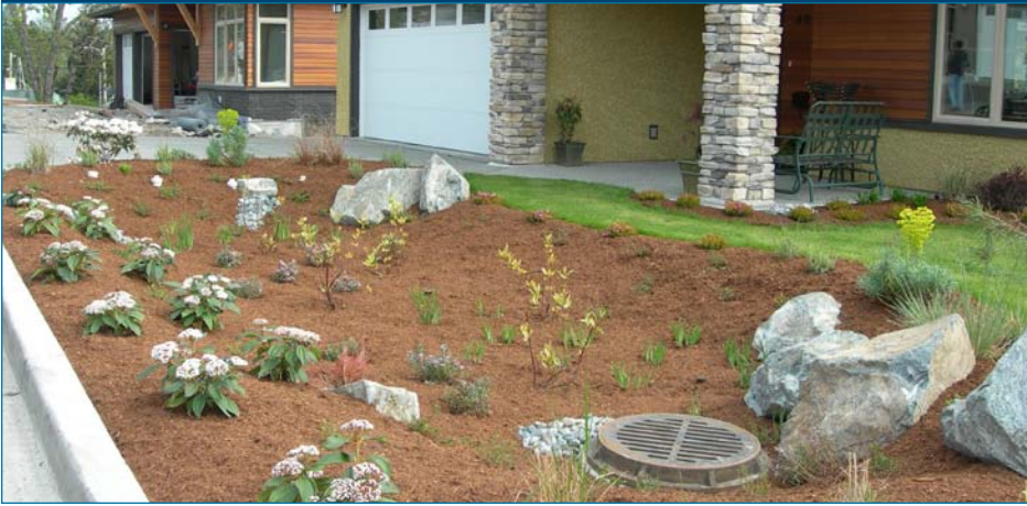
This newly planted rain garden will help reduce flooding while improving water quality.
