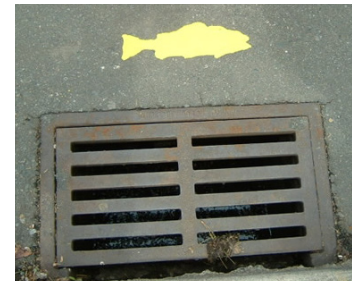
Storm drains connect directly to Bowker Creek and other urban waterways.
