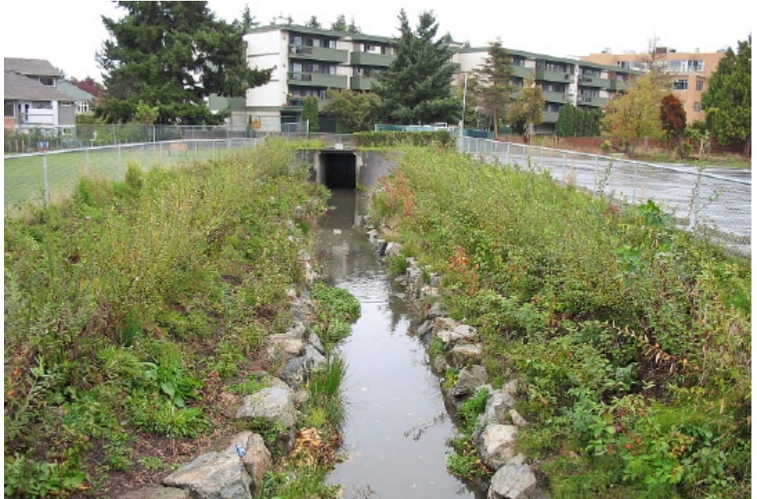
The restoration demonstration site (completed in 2005) at St. Patrick's elementary school fared well in 2006, even with unusual flooding events. PHOTO CREDIT: Tanis Douglas
