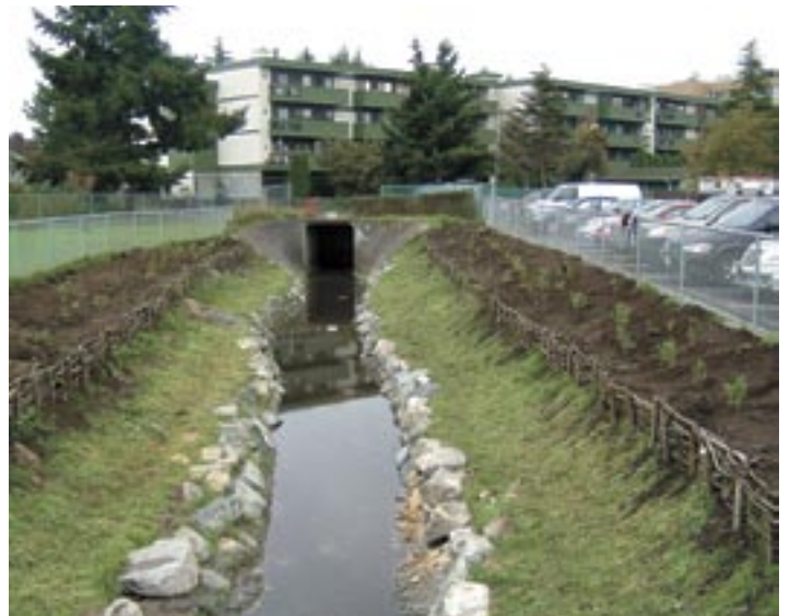
AFTER. Bowker Creek after bank stabilization, bioengineering and planting were completed.
