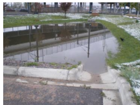
Figure 2 Infiltration basin located away from sewer pipes. Photo Credit: Construction Specifier Magazine
