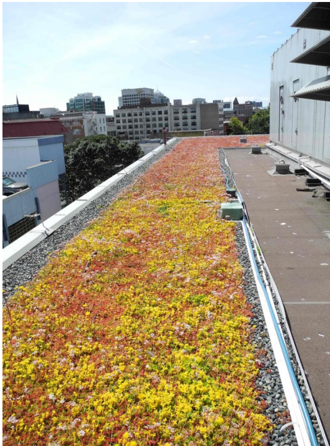
Figure 2 Extensive green roof, CRD Headquarters, Fisgard St., Victoria
