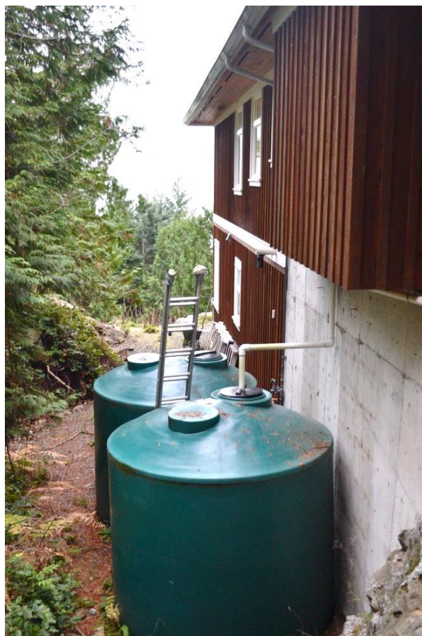
Figure 1 Cisterns capturing roof water for residential indoor and outdoor non-potable water use. Photo credit: Kim Stephens, Bowen Island, BC.
