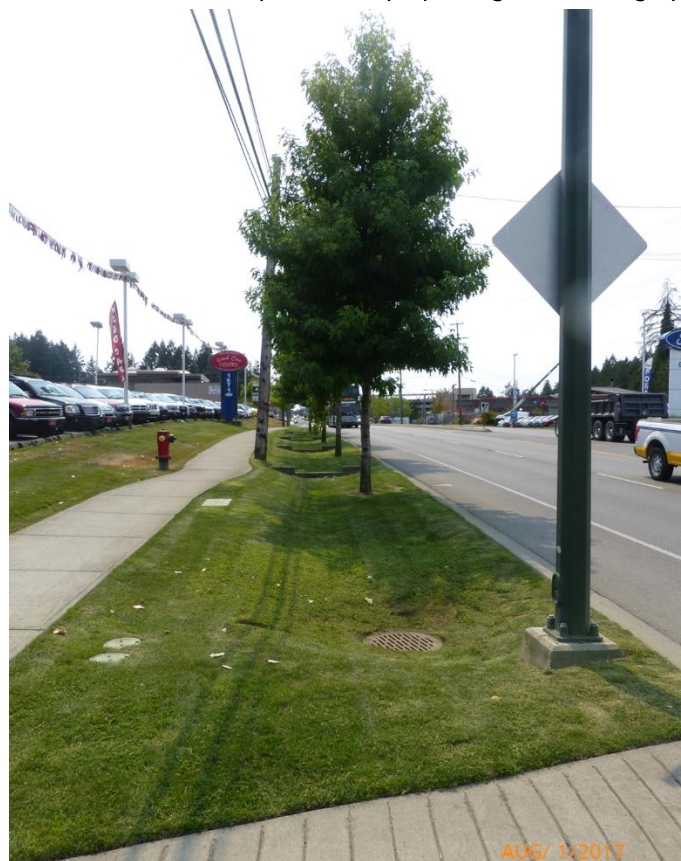
Figure 2 Grassy Swale, View Royal. Note: Flat over-flow drain may get blocked by debris, beehive style is recommended. Photo Credit: Town of View Royal
