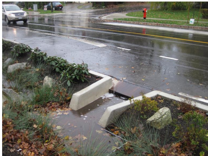
Figure 5 Curb example with steel flow dissipator
