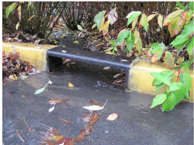
Figure 4 Steel curb inlet example
