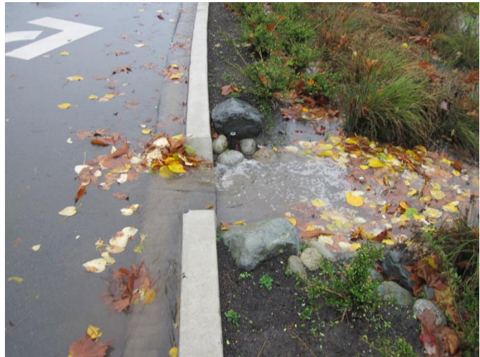
Figure 6 Curb cut example - Concrete curb let down with rocks
