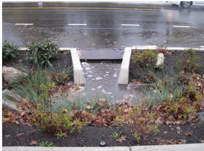
Figure 9 Vegetated Swale receiving runoff directly from road, Saanich
