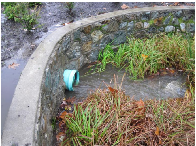
Figure 5 Stormwater inlet to rain garden, Saanich
