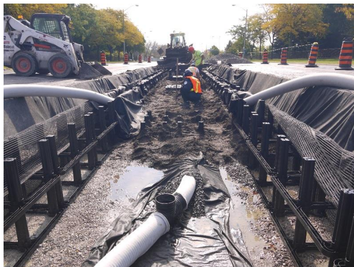
Figure 2 Same site under construction. Existing catch basin was retrofitted to direct stormwater into GSI facility with a distribution pipe (seen here) with soil cells and bioretention media. Photo Credit: Credit Valley Conservation
