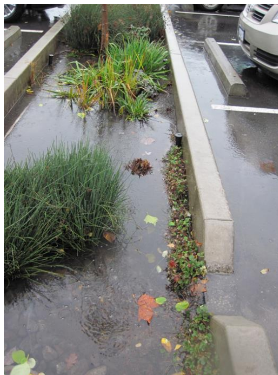
Figure 3 Sunken planter style, flat bottom rain garden in commercial area parking lot, Saanich
