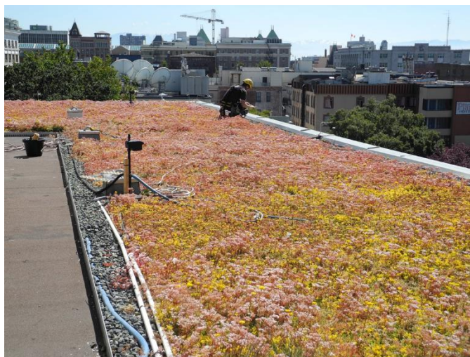
Figure 1 Extensive green roof, CRD Headquarters, Fisdard St., Victoria
