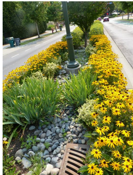
Figure 3 vegetated infiltration traffic island, Island Highway, View Royal. Photo Credit: Town of View Royal
