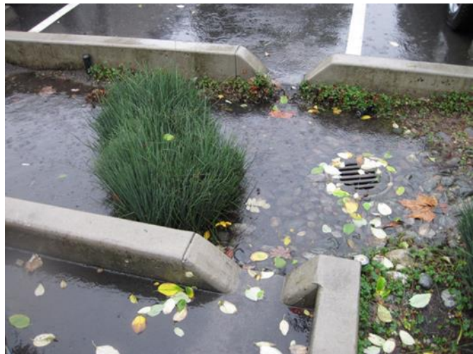
Figure 2 Flat drains such as in the infiltration planter can easily get clogged with leaves
