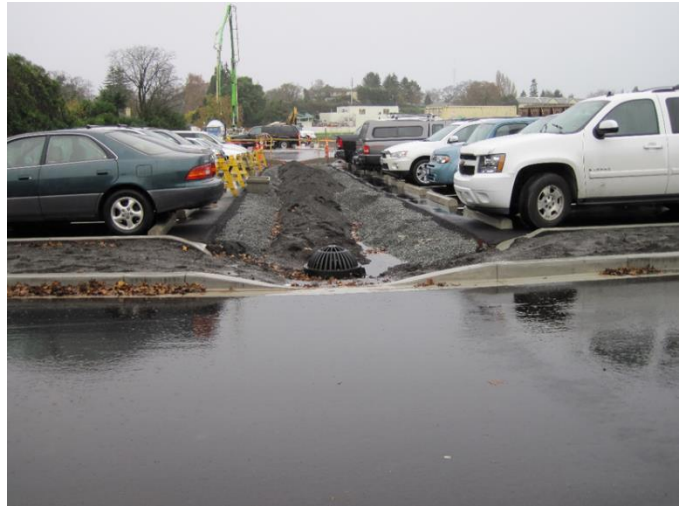
Figure 10 Swale under construction at Oak Bay High School parking. Raised or beehive style grates are recommend.
