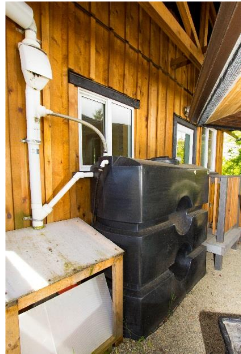
Figure 3 Cistern collecting roof water with pump (covered to the left) pumping collected roof water to the garden. Photo Credit: Victoria Compost Education Centre
