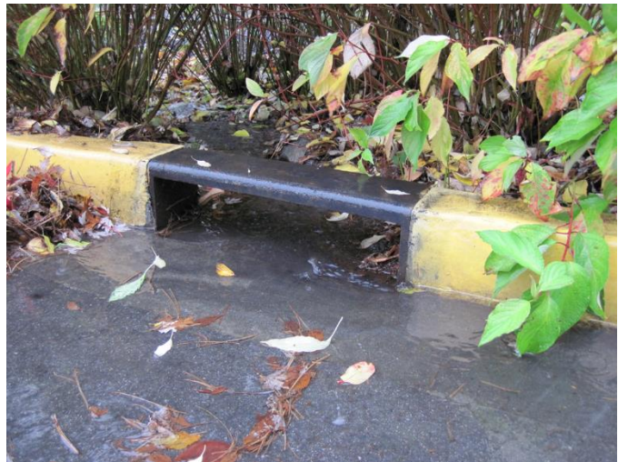
Figure 4 Inlet type for rain garden with no dissipater
