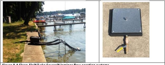
Figure 9.4 Clean-Flo™/Lake Savers™ laminar flow aeration systems
