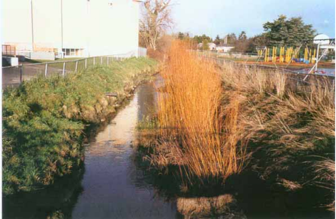
PLATE 1: Zone 1 of Bowker Creek adjacent to St. Patrick School showing eroding west bank and golden willow growth in channel at base of east bank.
