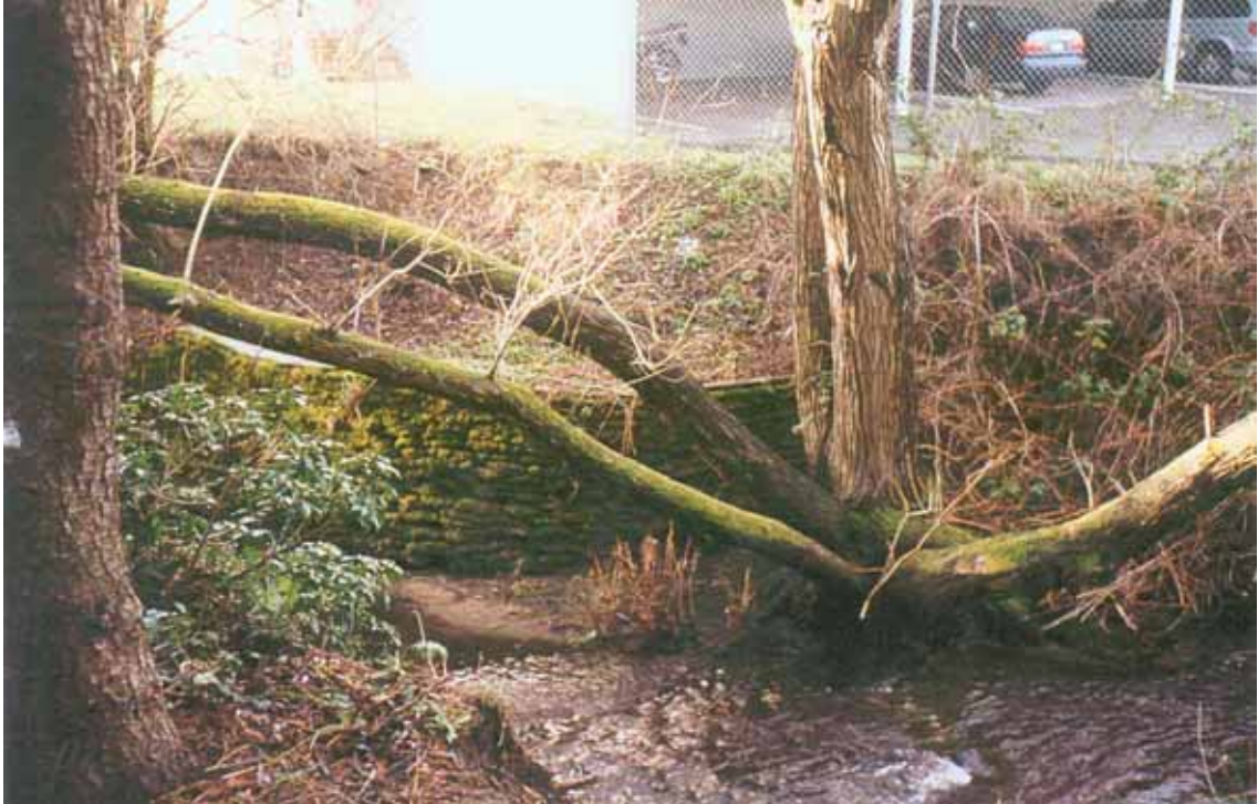
PLATE 7. Zone 5 of Bowker Creek showing cement filled sand bags and mature golden willow growth on west bank adjacent to apartment building complex.
