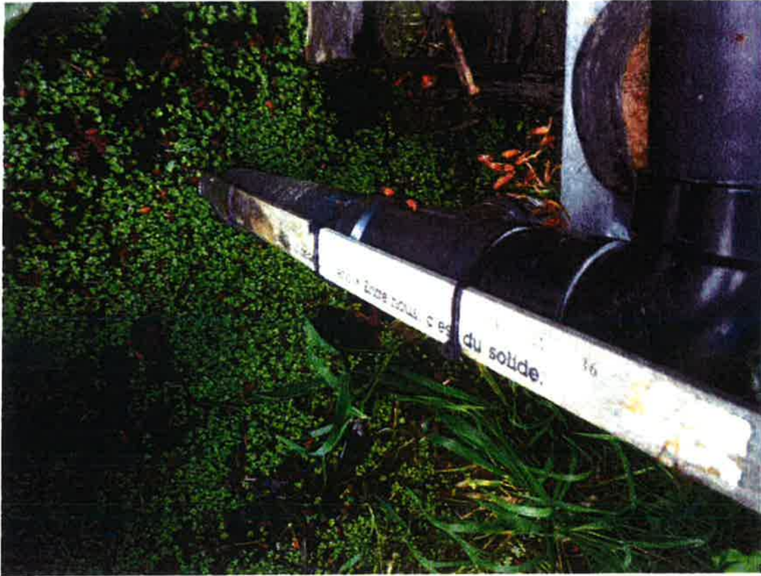
Gardom Pond Reservoir Water Level Gauge – To be replaced at suitable location.
