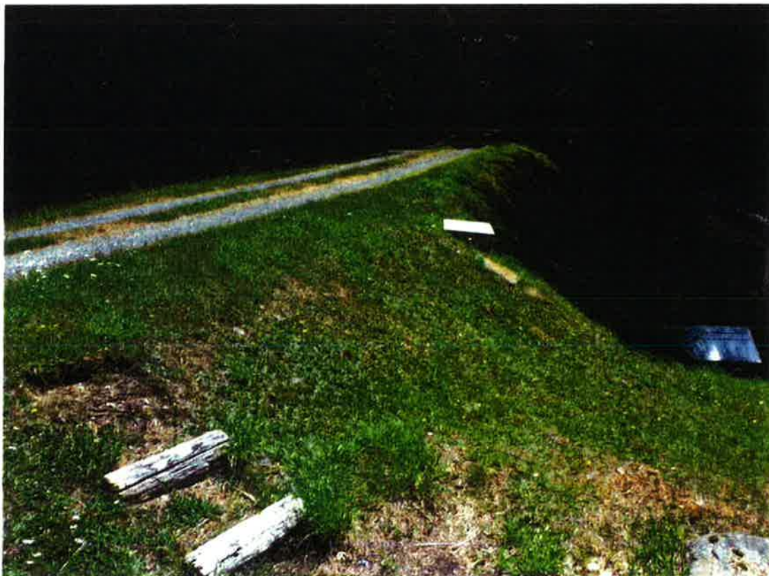
Gardom Pond Dam – Downstream face
