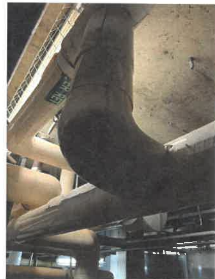
Isolation Valve Insulation Compromised and Causing Pipe corrosion.
