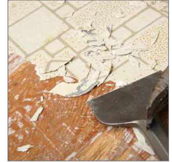
RENOVATION WASTE (residential)
