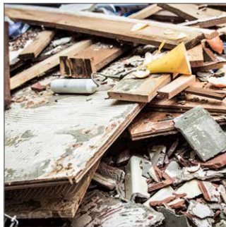
SAFE RENOVATION WASTE DISPOSAL
