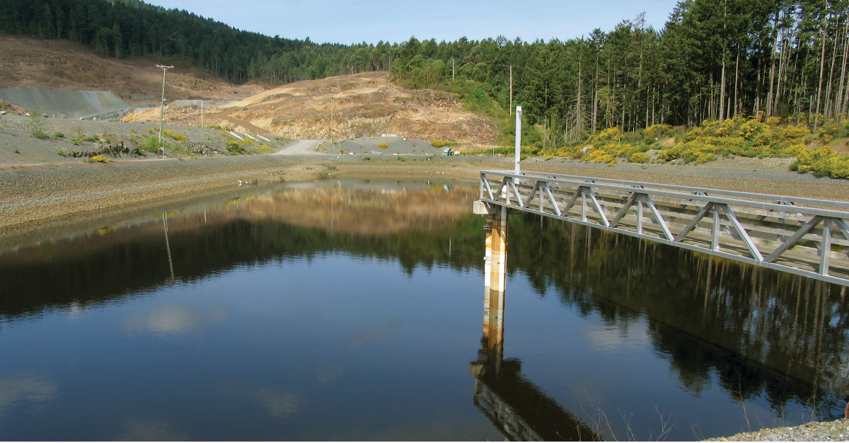
Leachate lagoon at Hartland landfill.
