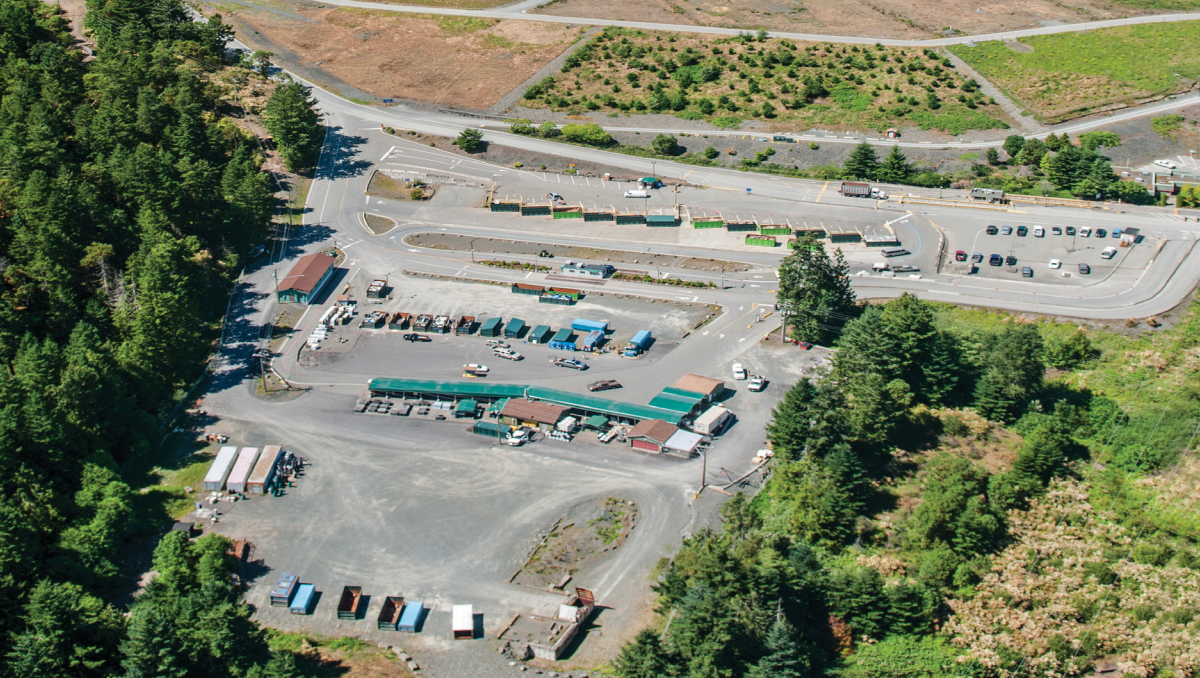
Front end section of Hartland public drop off area
