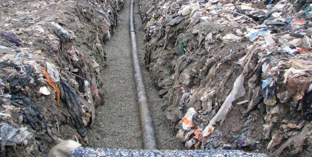
Installation of landfill gas collection piping at Hartland
