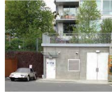
VICTORIA BC – Dockside Green WWTP, Capacity 0.19 MLD existing, 0.38 MLD with additional membrane filters
