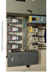
Figure A-19 Existing WTP Pump Control Panel
