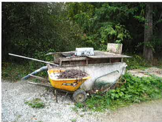
Current receiving station: manual screen cleaning.
