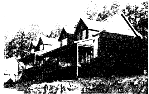
Existing Built Form Example
