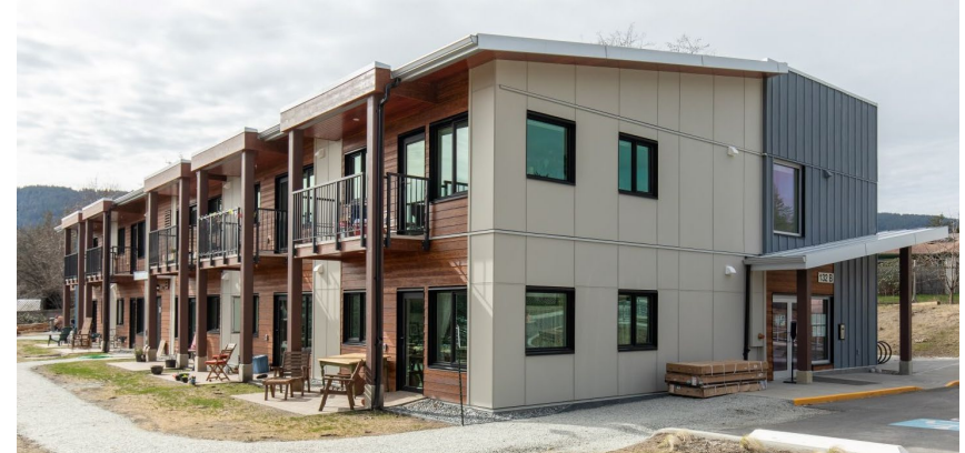
Phase II: 22-Units
