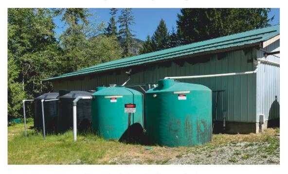
Figure J. Rainwater Storage Tanks
