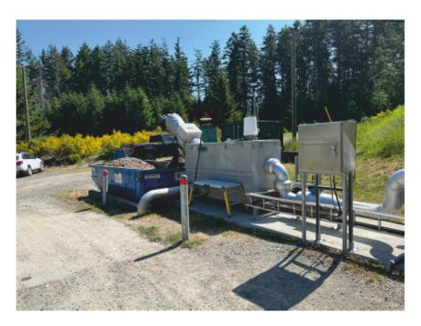
Figure F. Waste-Stream Receiving Grit Removal and Screening Facility
