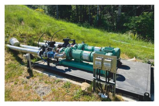
Figure H. Storage Tank Recirculation Pumps
