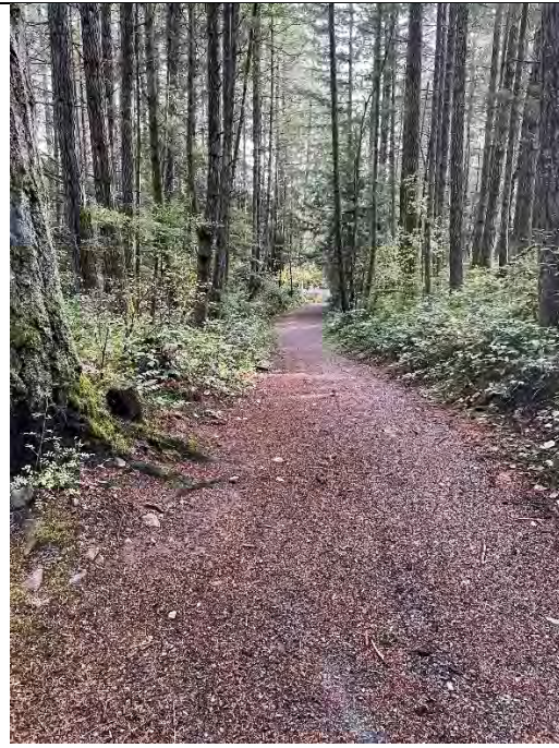
Long Segment of Trail with Steep Grade (10-15%) is a Barrier to Visitors with Mobility Constraints
