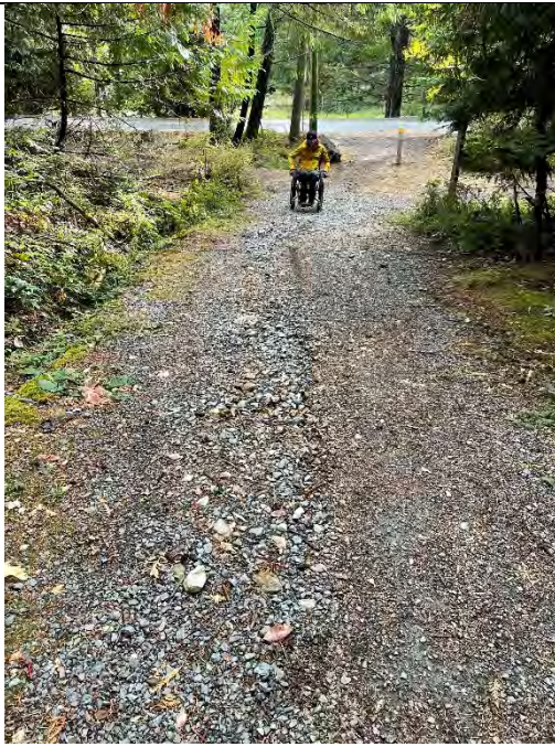
Erosion Channels in Steeper Segments of Trail Expose Base Materials and Create Barriers
