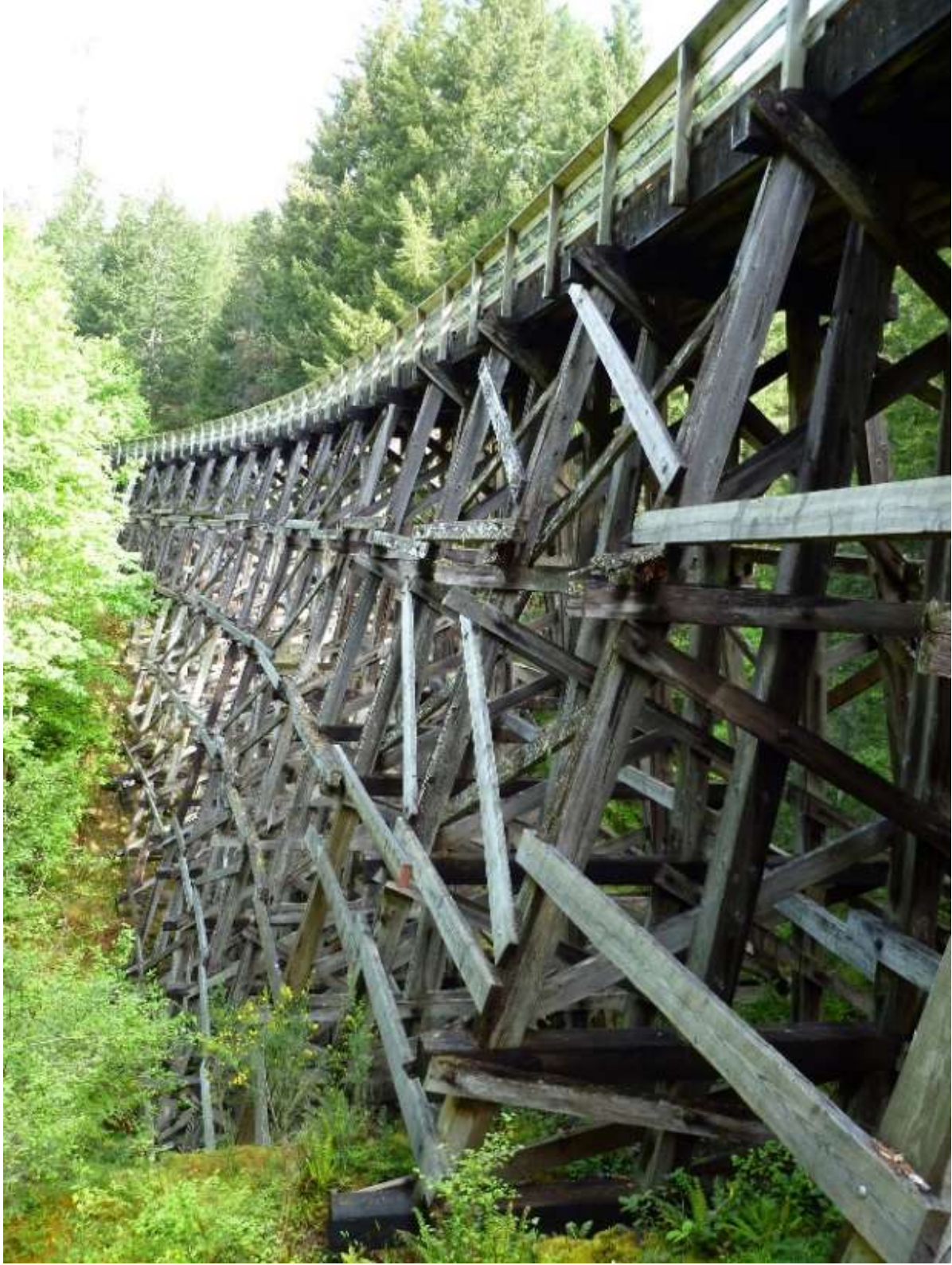
Todd Creek Trestle – Looking North
