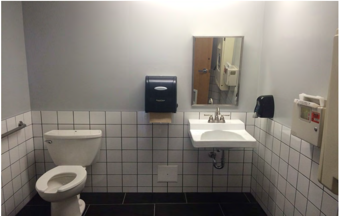
Repairs and upgrades of Panorama washroom
