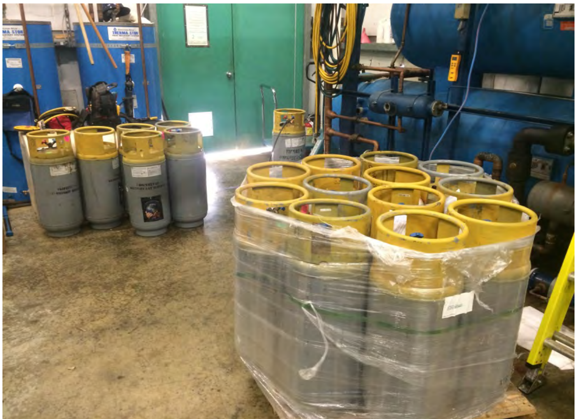
Refrigeration plant Freon removal
