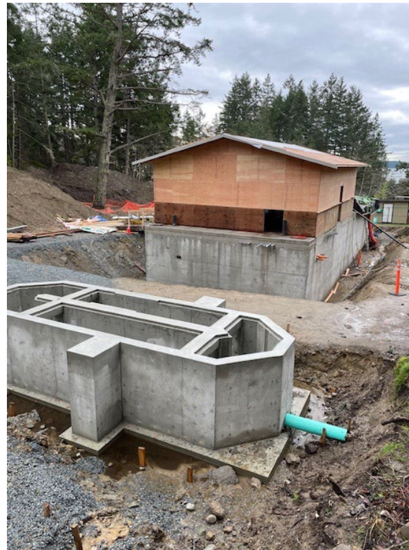
WWTP Tanks and Operation Building
