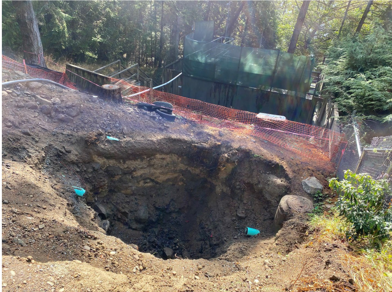
Excavation at Cannon Pump Station
