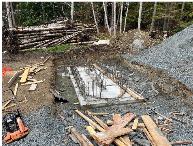
Inlet Screen Channel Foundation
