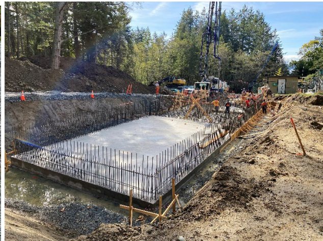
Pouring concrete for WWTP Tanks
