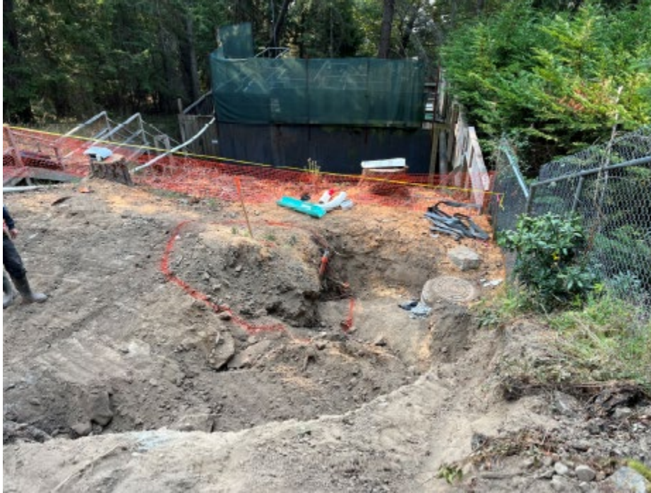
Excavation at Cannon Pump Station
