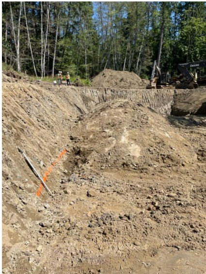
Rock at Schooner WWTP
