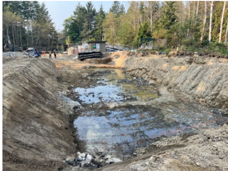
Rock Removed and Excavation Complete
