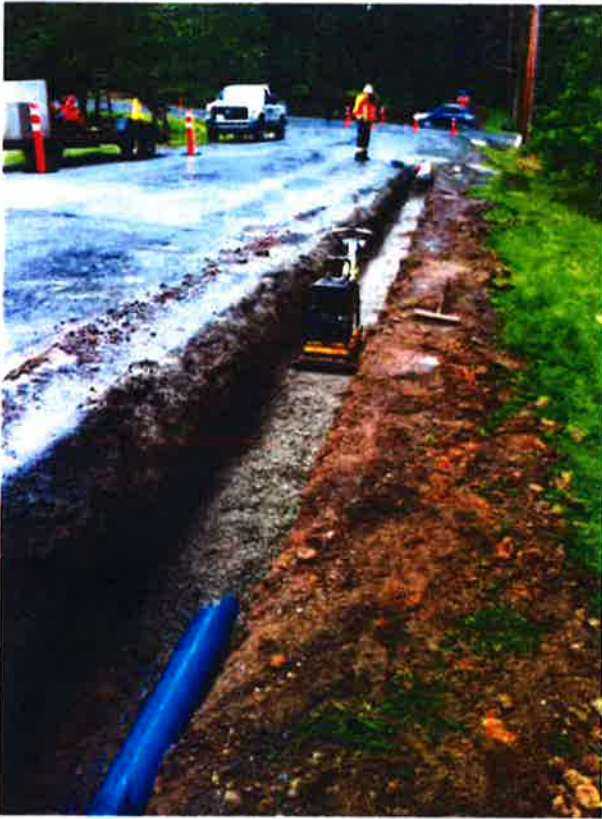
Photo: Water main installation
