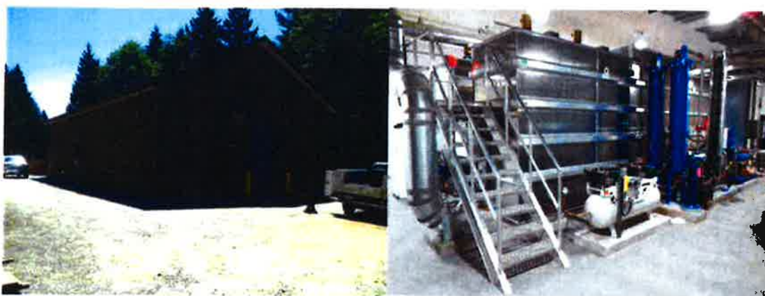
New Water Treatment Plant Building at 47284 Schooner Way
