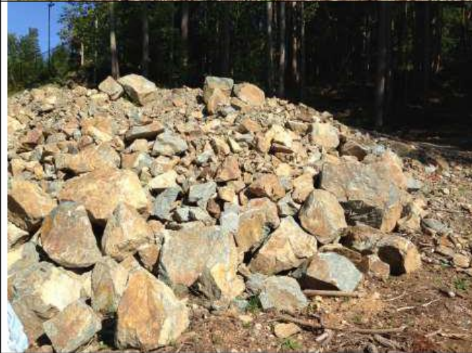
Shotrock/boulder fill at east end of the roughed-in driveway
