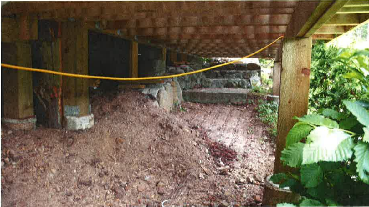
Photo 5. New deck was built over top of old stairs and pathway.
