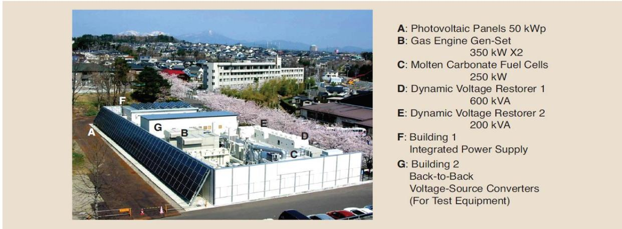
Figure 5 – The Sendai Microgrid at Tohoku Fukushi University [27]
