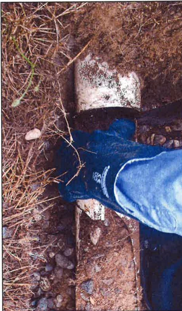
Cracked septic system pipe being removed.
