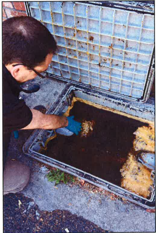
Source control staff inspecting a grease trap.
