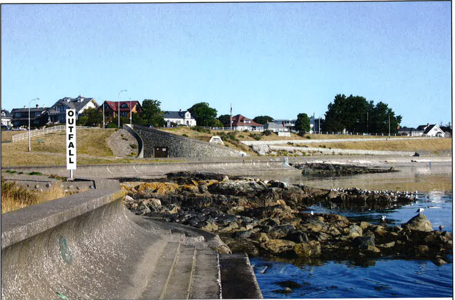
Outfall at Clover Point.
