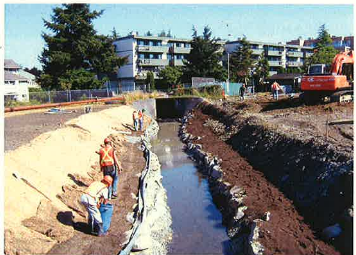
Applying erosion control fabric and seeding the banks of Bowker Creek.
