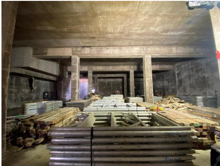
Arbutus Attenuation Tank
