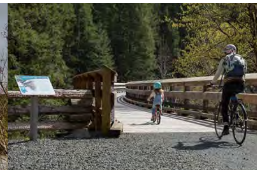
Todd Creek Trestle
