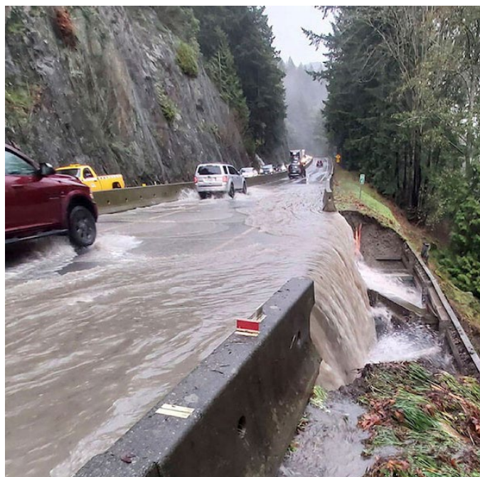
Malahat washout during November 2021 extreme rain event (Credit: Emcon Services Inc.)
