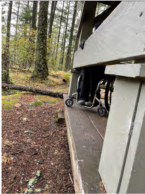
Pavilion Does Not Include Wheel Stops Which Poses a Tipping Hazard
