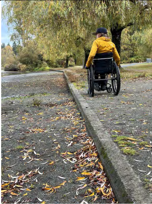
Concrete Transition to Beach is a Barrier
