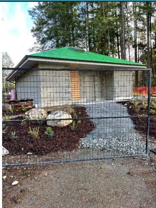
Grades to Toilet Building May Make Access Difficult
