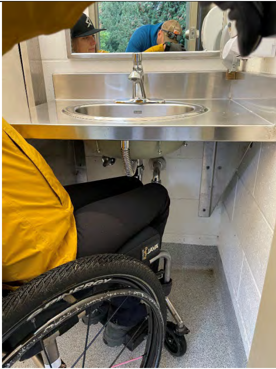
Limited Access to Approach Sink
