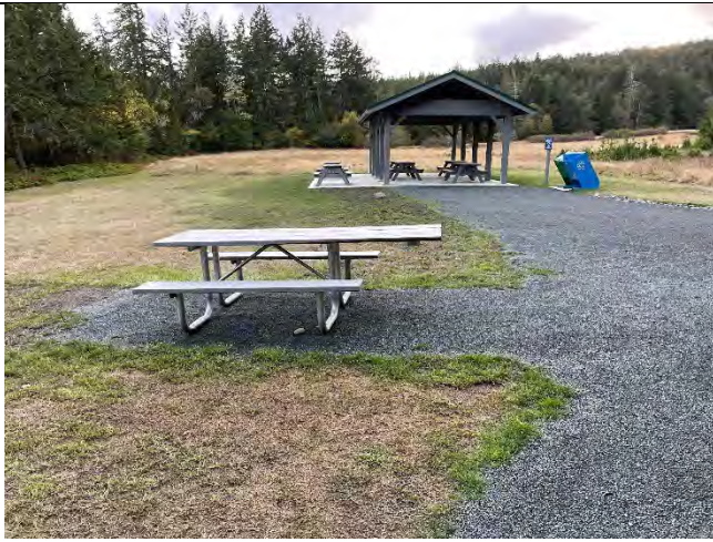
Surfacing Around Picnic Table Limits Ability to Travel Around Table & Accessibility Overhang on One End Limits Visitor Choice
