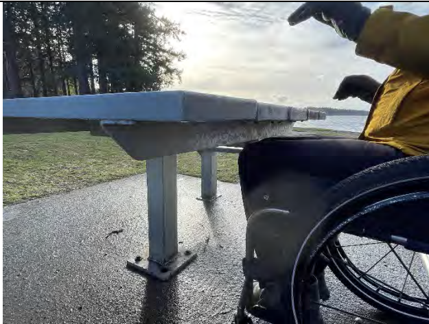
Installation Orientation Limits Ability to Approach Under Table
