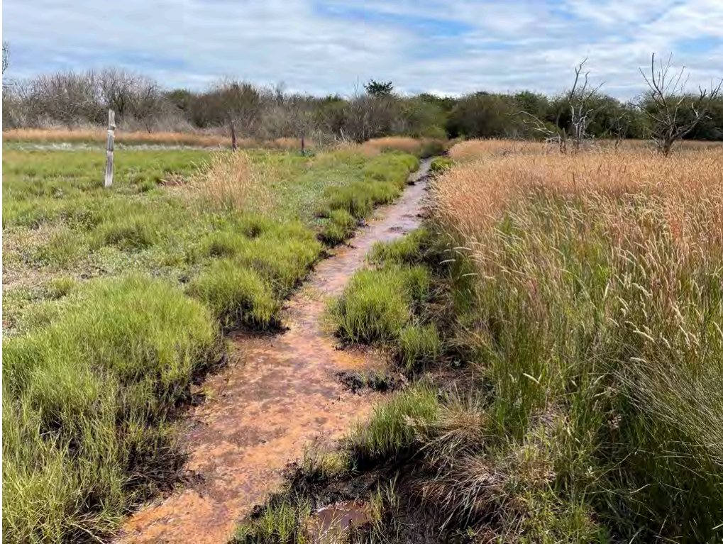
Ditch 5 July 16, 2022. Taken from mid-point of channel looking east.
