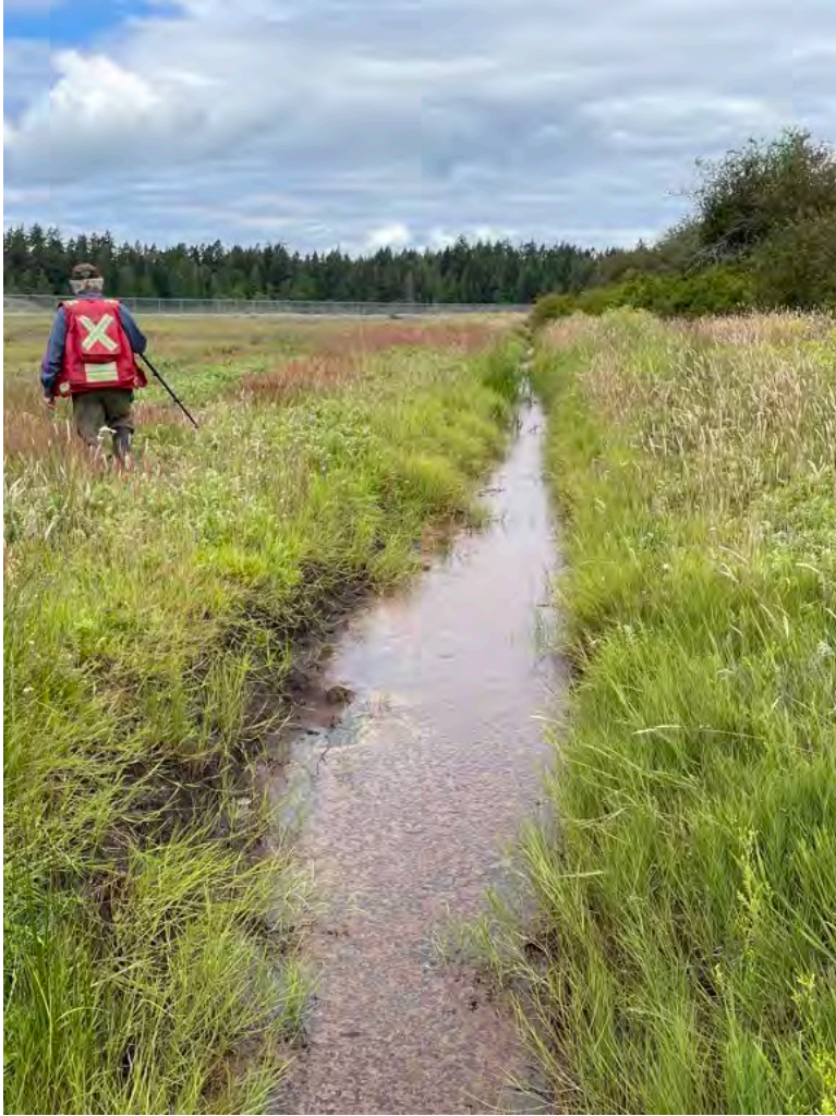
Ditch 2 from middle of the channel looking northwest July 16, 2022. The channel is more open and was draining well.
