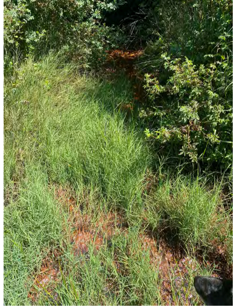
Confluence of Ditch 2 and Ditch 3 July 5, 2021.
