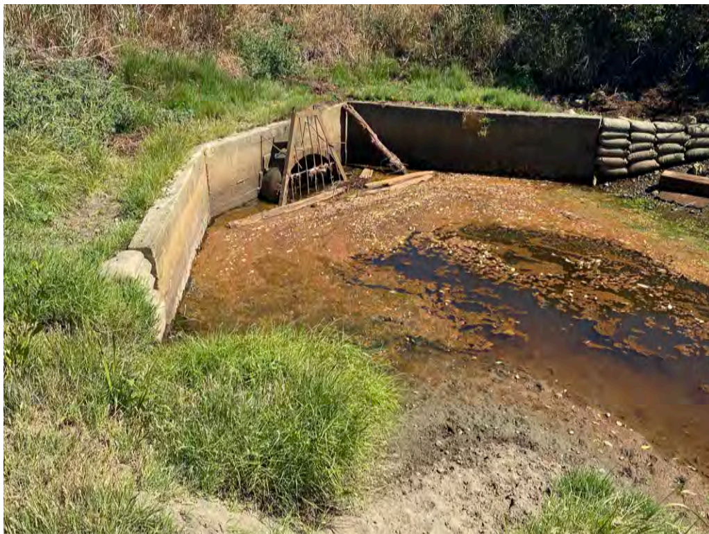
Trash rack upstream of the tide gate July 5, 2021.
