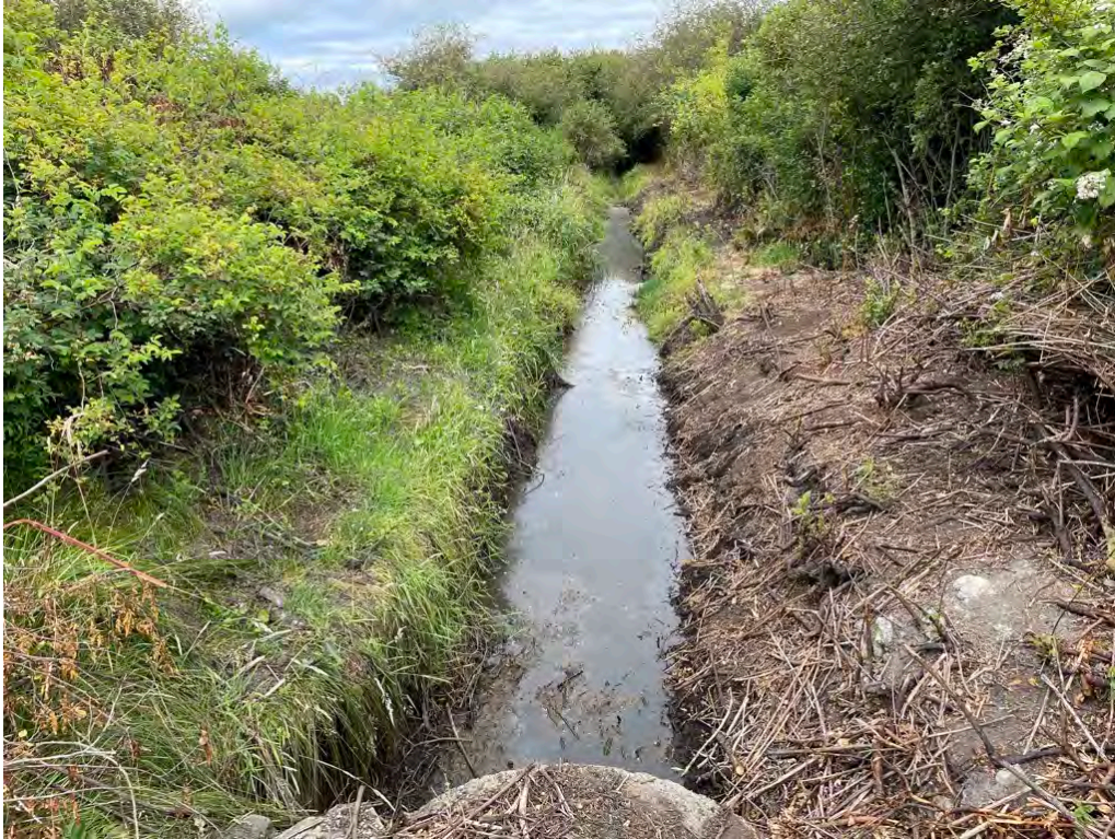
Looking north from trail crossing over intersection of Ditches 3 & 4 looking north up Ditch 3, July 16, 2022. The lack of vegetation along the channel may encourage new growth in the channel as light is no longer limited.
