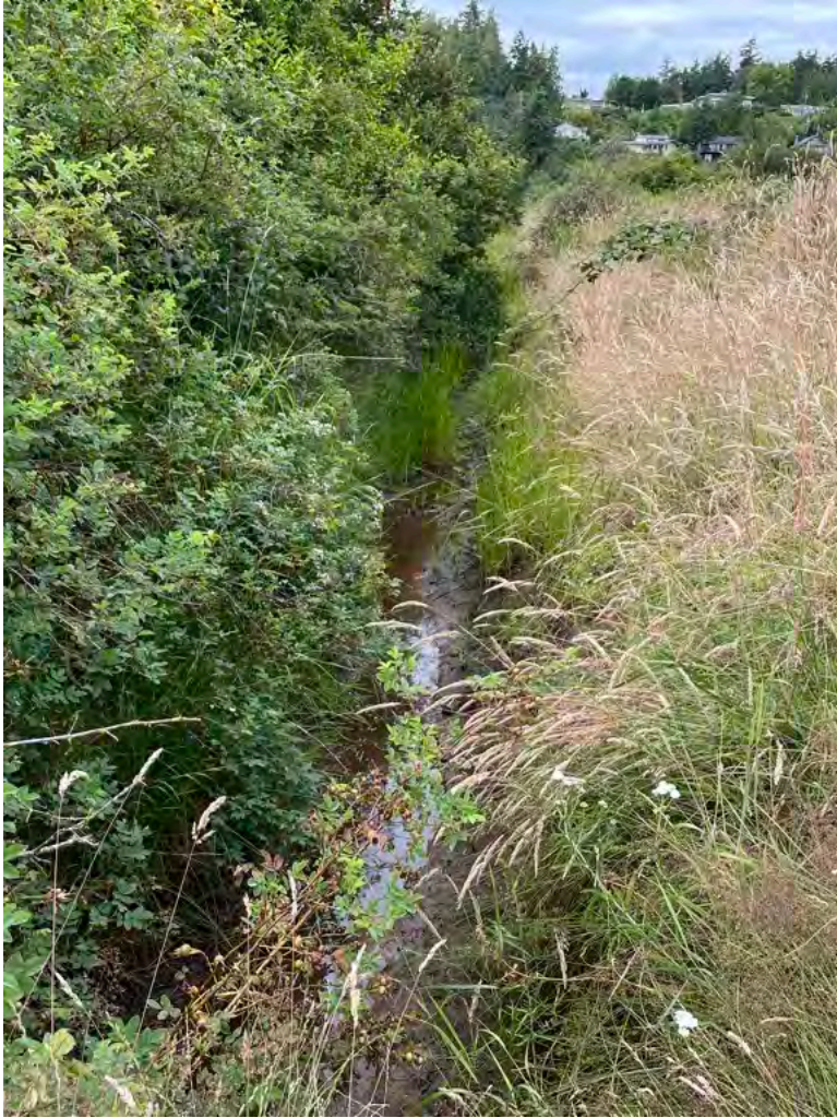
Lamont ROW ditch looking west, downstream end July 16, 2022. There was a very small amount of water in the channel and positive drainage was observed.
