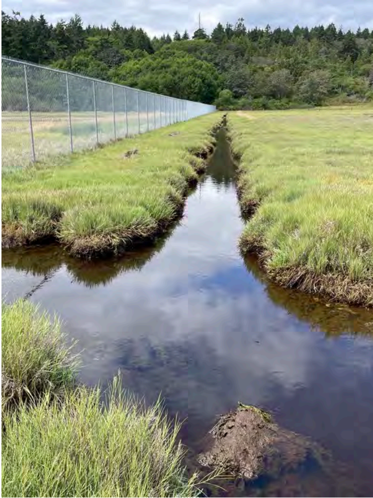
Ditch on Tsawout land running east-west along chainlink fence (looking west) July 16, 2022.
