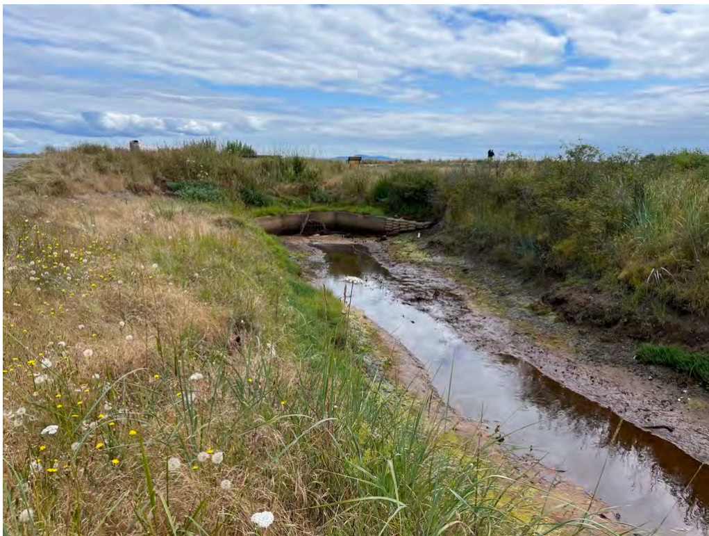
Lamont ROW at the trash rack upstream of the tide gate July 16, 2022.
