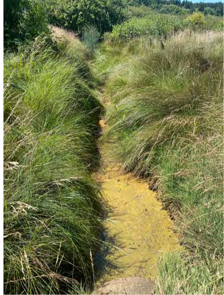
Downstream end of Ditch 1 July 5, 2021.
