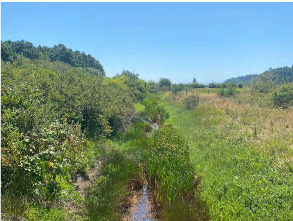
Campground ditch July 5, 2021 prior to 2021 maintenance.
