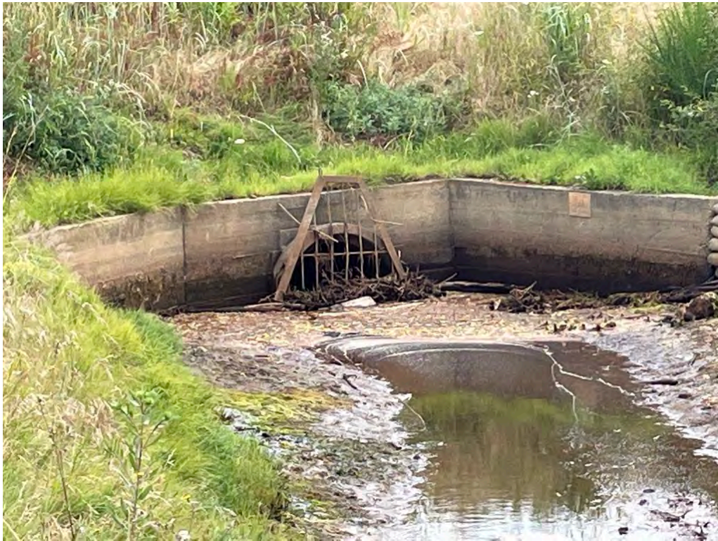
Trash rack upstream of the tide gate July 16, 2022.
