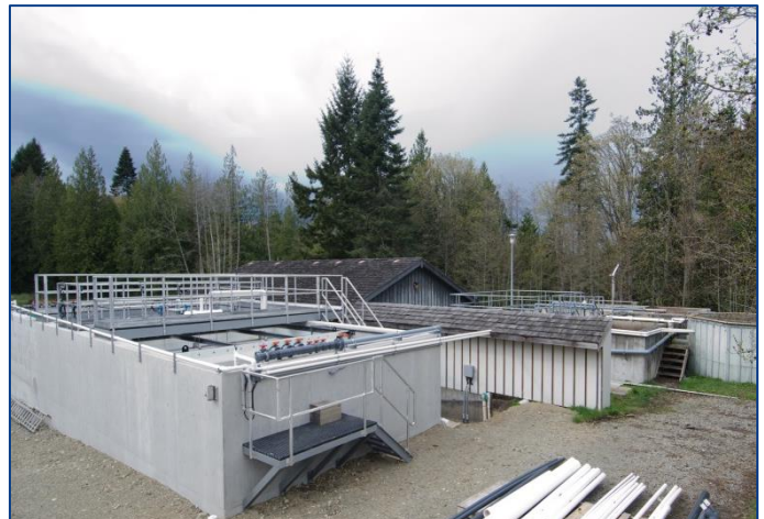
Mill Springs Village WWTP, BC
