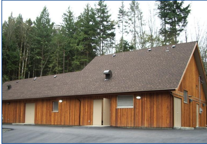
Nanoose First Nation WWTP, BC
