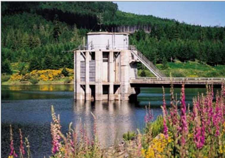
The intake tower at the Sooke Reservoir.
